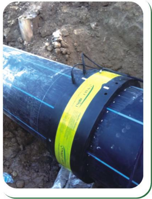
1400mm Electrofusion Coupler Site Installation
